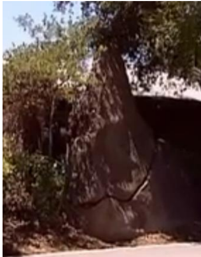
2010 Photo of Victoria Rock with its large crack
